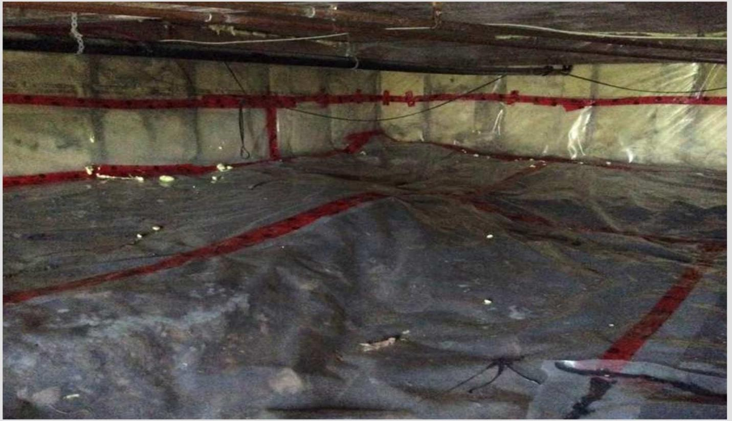
Above: Adding insulation to the crawlspace walls and poly on the ground to stop the moisture in Fort Albany.
