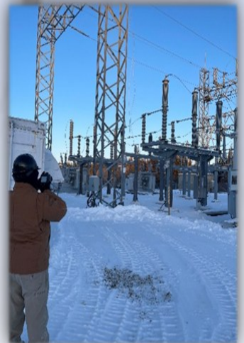
Simon performing infrared camera inspections at connection points on high voltage equipment.
