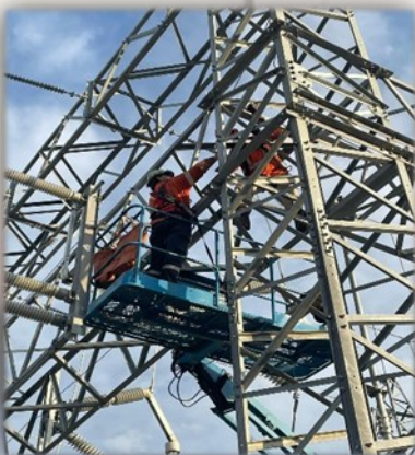
Power North crew upgrading steel structure for bus isolation project
