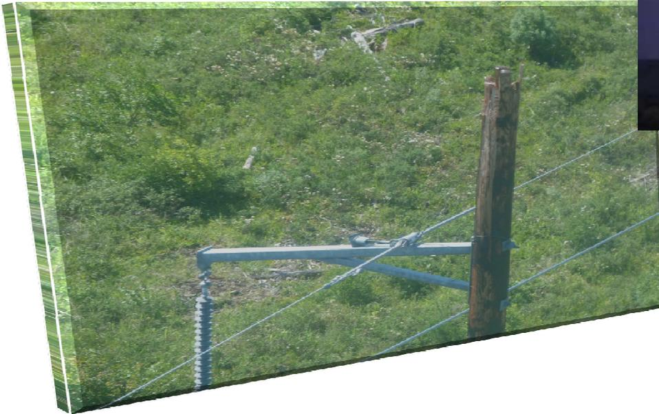
One of the thunderstorms lightning strikes spliced the pole tope on the line going from Moosonee to Kashechewan. The sky wire also carrying internet for all three communities was ripped off the pole and landed on the crossarm it is temporary held by ground wire in safe position. The repairs is planned for the winter road season when the area is accessible for the bucket truck.
