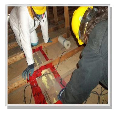
Above: Air sealing an attic floor in Kashechewan in preparation for blowing in insulation.
