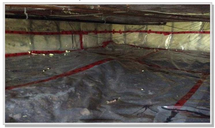
Above: Adding insulation to the crawlspace walls and poly on the ground to stop the moisture in Fort Albany.
