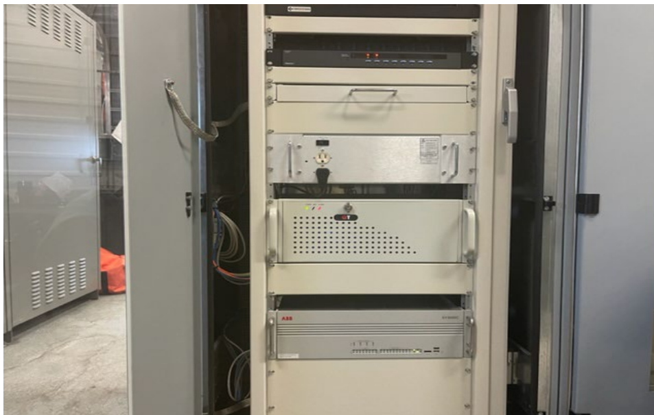
4 Picture Above: One of two servers replaced the top server is existing and the bottom is the new 5 server
